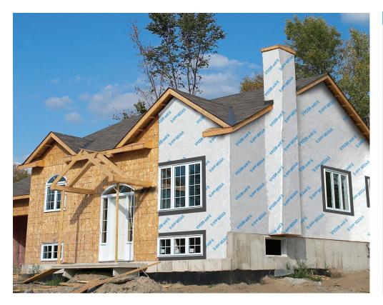
VYCOR® enV-S™ sheet-applied, self-adhered weather resistive barrier provides exceptional protection against water damage and air infiltration. It helps preserve the home's structural integrity and contributes to improved energy efficiency.
