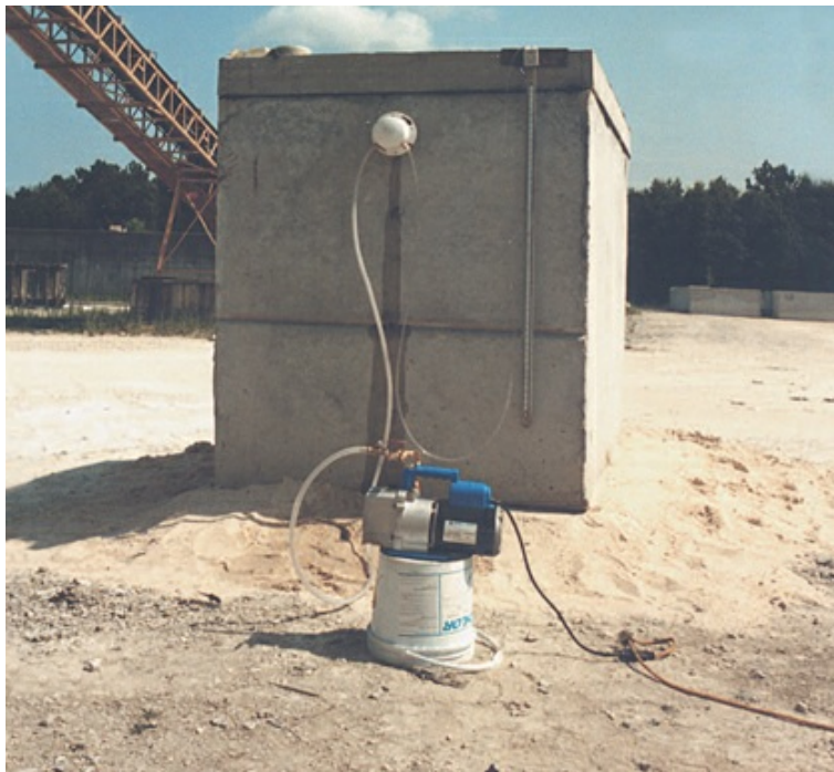
Vacuum testing of concrete septic tanks
