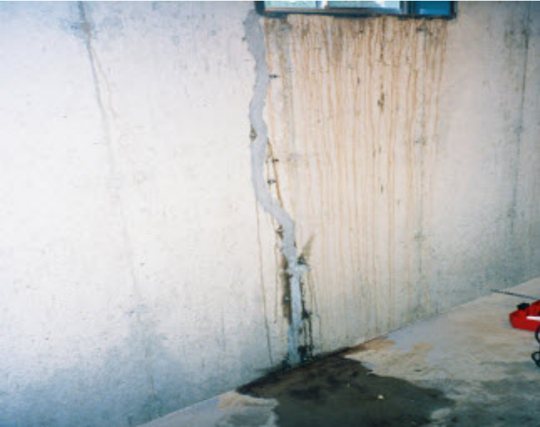
Figure 2. To drill at a 45° angle, drill distance must be 1/2 the thickness of the wall. EX. 12 inch thick wall = drill holes 6 inches from crack
